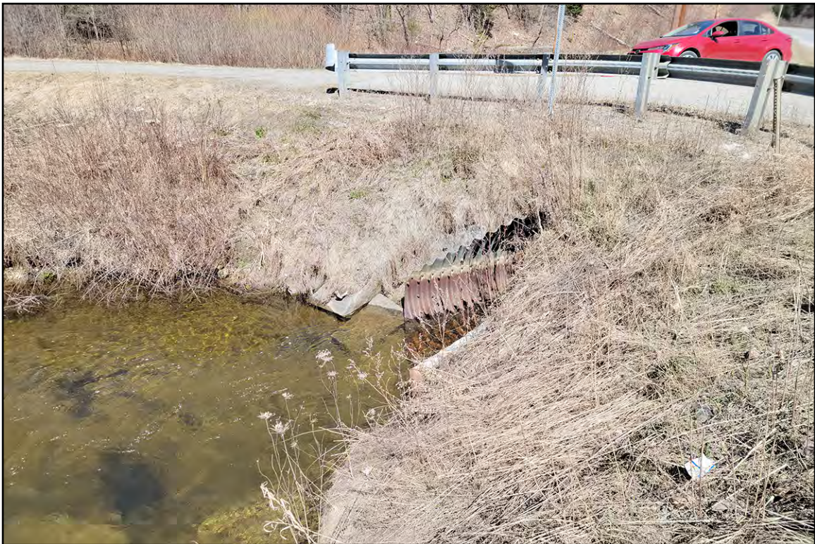
PLATE 2: Coventry Culvert No. 132, Facing Northwest
