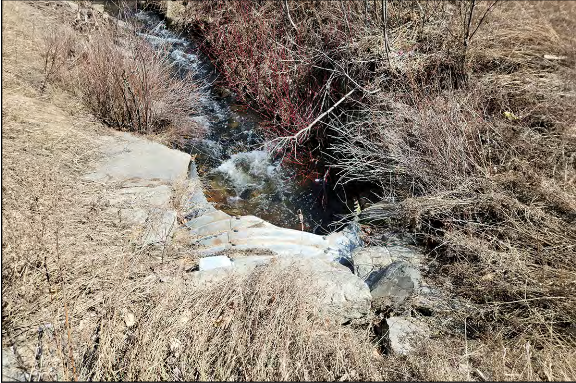
PLATE 2: North End of Culvert with Modern Ditch Used to Direct Stream/Runoff Water, View East
