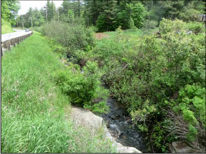
Figure 1. Stoney Bk above VT RT 14 pipe arch
