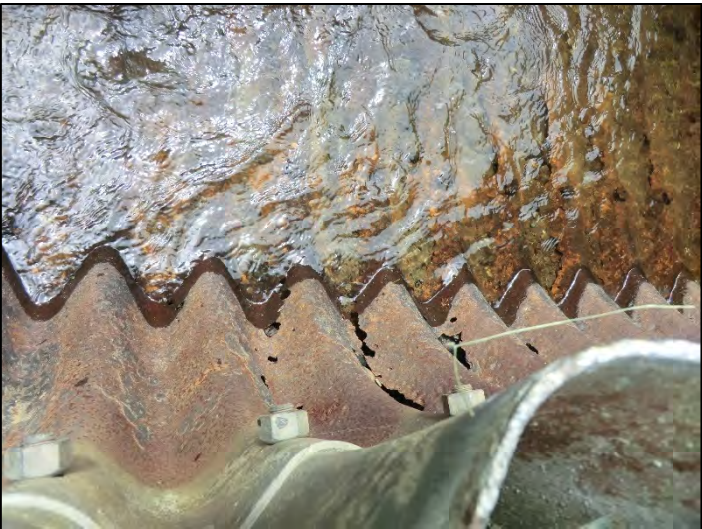
Figure 3. Deteriorated VT Route 14 culvert inlet
