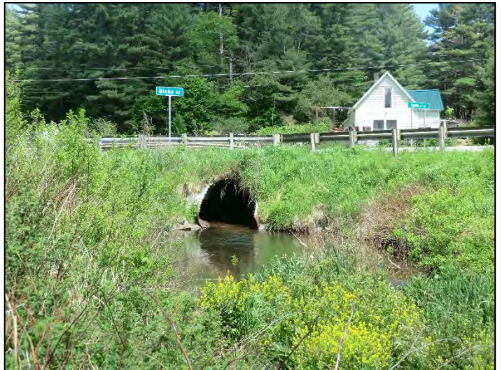
Figure 4. VT Route 14 culvert outlet
