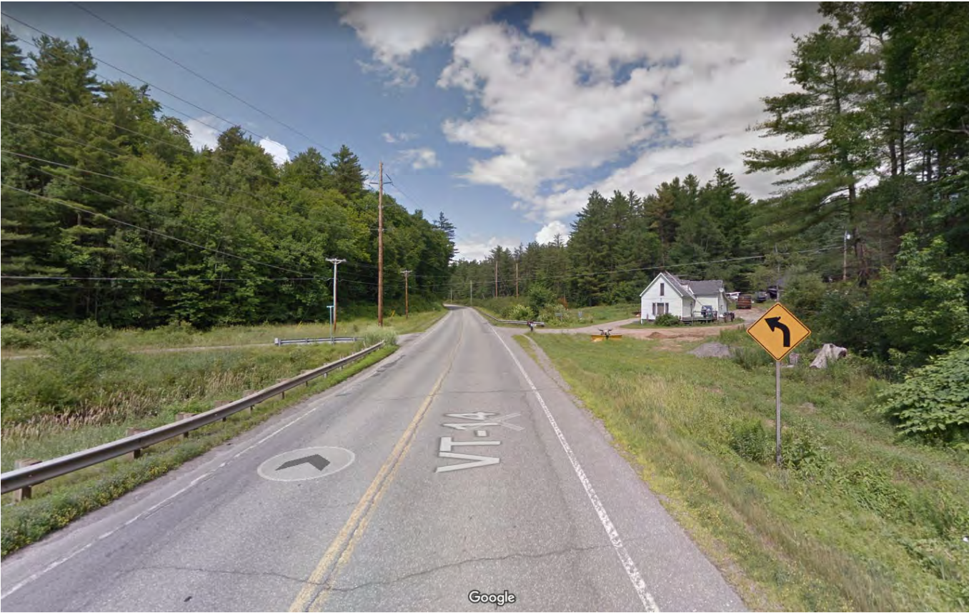
Looking north overt bridge 132
