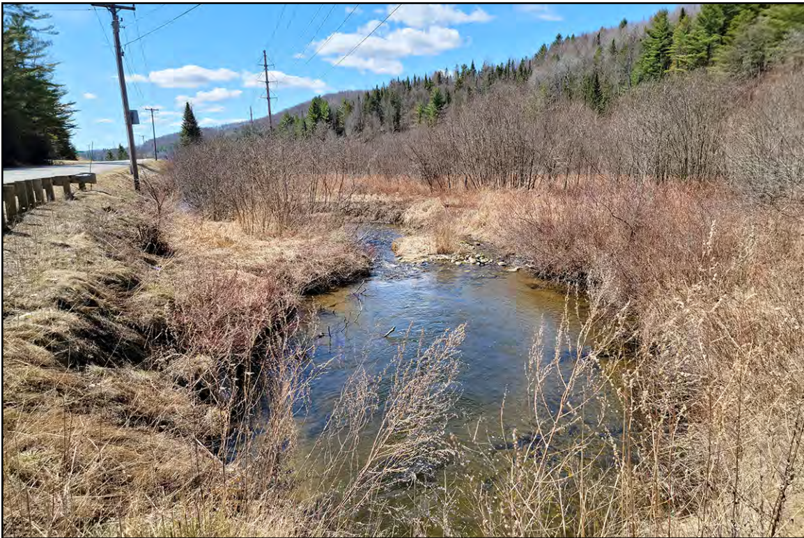
PLATE 3: South End of Culvert with Possible Stream, View South
