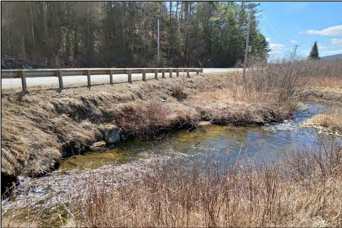
PLATE 1: Built-up Roadway Going Over Culvert, View South
