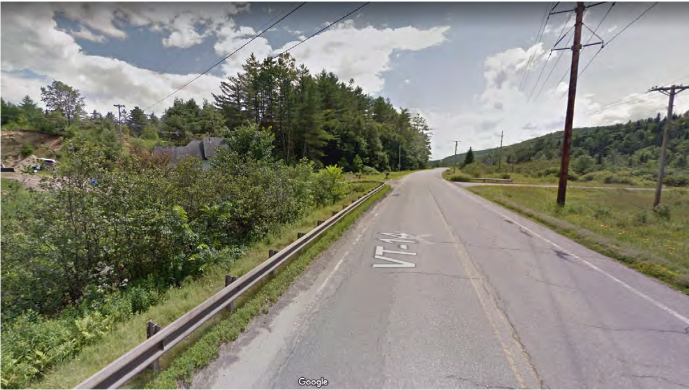
Looking south over bridge 132
