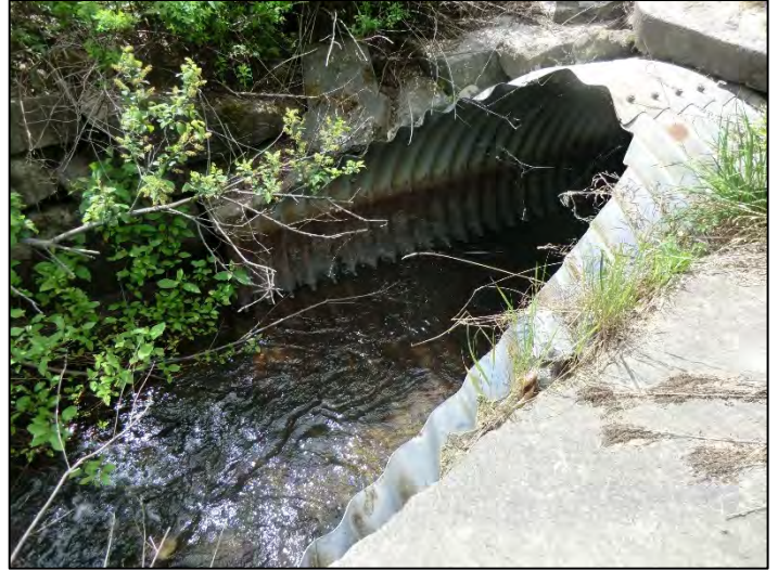
Figure 2. VT Route 14 culvert inlet
