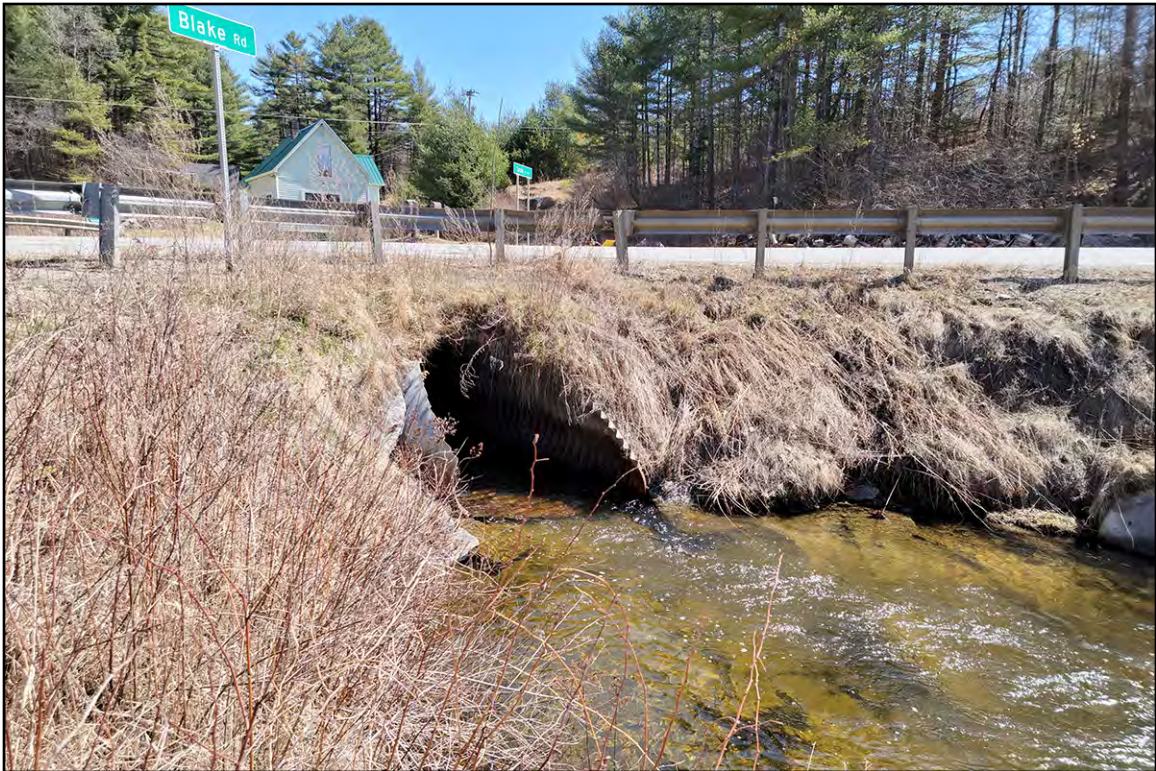
PLATE 3: Coventry Culvert No. 132, Facing Northeast
