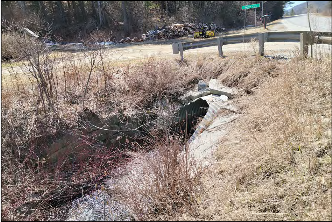
PLATE 1: Coventry Culvert No. 132, Facing South
